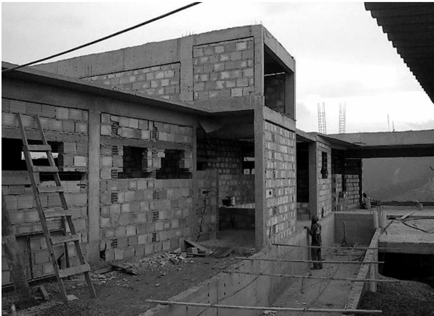
Figure 2.3 An Expensive House under Construction with Precisely the Same Technology as the Favelas
